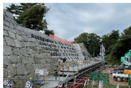
Restoration construction site
